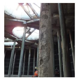
Fig. 8: Example of damaged column under the hot water basin, prior to concrete repair.
