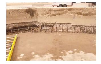
Fig. 12: Concrete repairs at the wall-to-floor cold joint in the cold water basin.
