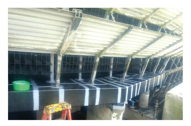
Fig. 9: Previously repaired beams strengthened with CFRP.
