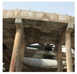
Fig. 2: Leaking joints in precast concrete hot water basin led to deterioration throughout the concrete structure.
