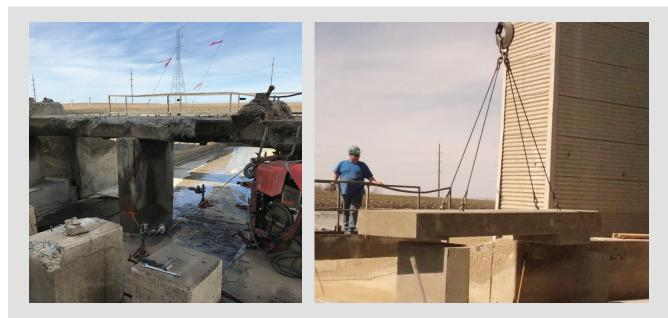
Fig. 11: Severely deteriorated beam was wire cut, removed and replaced with new freeze-thaw resistant precast beams.
