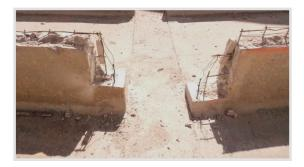
Fig. 3: Prepared precast fins with Type 1A galvanic anodes awaiting new high performance concrete.
