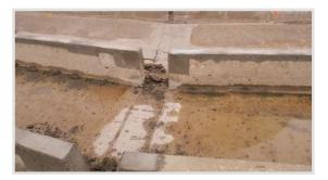
Fig. 4: Concrete fins repaired, prior to protective coating application.
