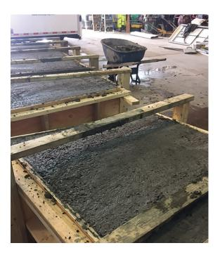
The same strengthening technology was expected to be used on Tower #91 however advanced deterioration was discovered during the fall inspection. Based on this new information, it was decided to completely replace the severely deteriorated precast beam that spanned the outlet flume. Based on the relatively short shutdown schedule, utilizing precast concrete was deemed to be the most effective approach to replace the roughly 24'x4'x1.5' beam.
