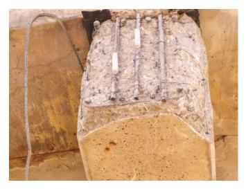
Fig. 7: Deteriorated beam end with concrete removed and Type 1A embedded galvanic anodes installed.
