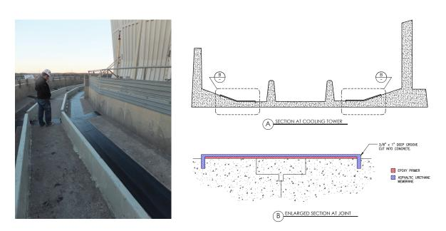
Fig. 5: Completed hot water basin floor repairs including concrete repairs and waterproofing.
