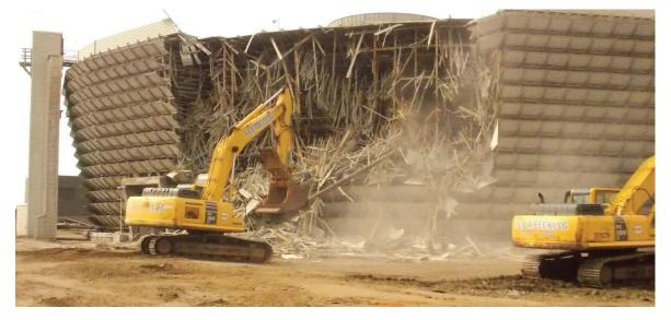
Fig.1: Demolition of the outer structure of the cooling tower to expose the interior concrete structure.
