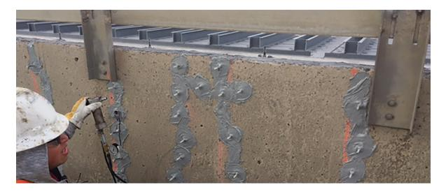
Fig. 6: Epoxy adhesive injected to seal fine cracks in the basin walls.
